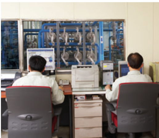
[Thermal Energy Storage System]
